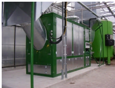
2G-Cenergy is marketing its high-efficiency 2G biogas CHP cogeneration system in the U.S., where it can be applied with other renewable energy technologies at landfills and wastewater treatment facilities. PHOTO: 2G-CENERGY
