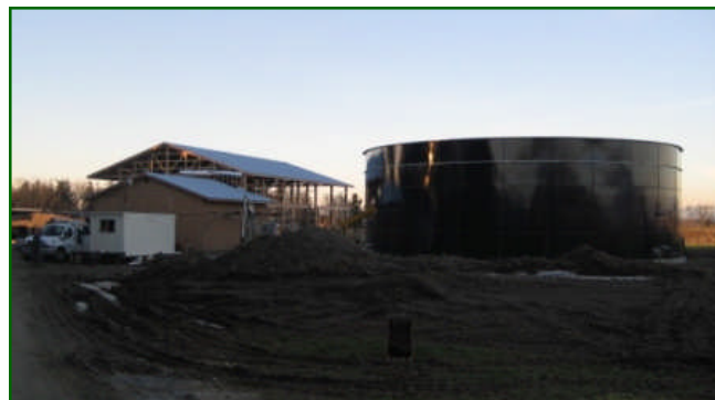
The DARITECH Anaerobic Digester at the VanDyk Dairy Farm in Lynden, WA (above). 2G's agenitor ® 212 has been placed inside the Customers Power House (left).
