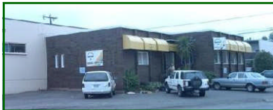
RDI Headquarter in Seattle, WA
